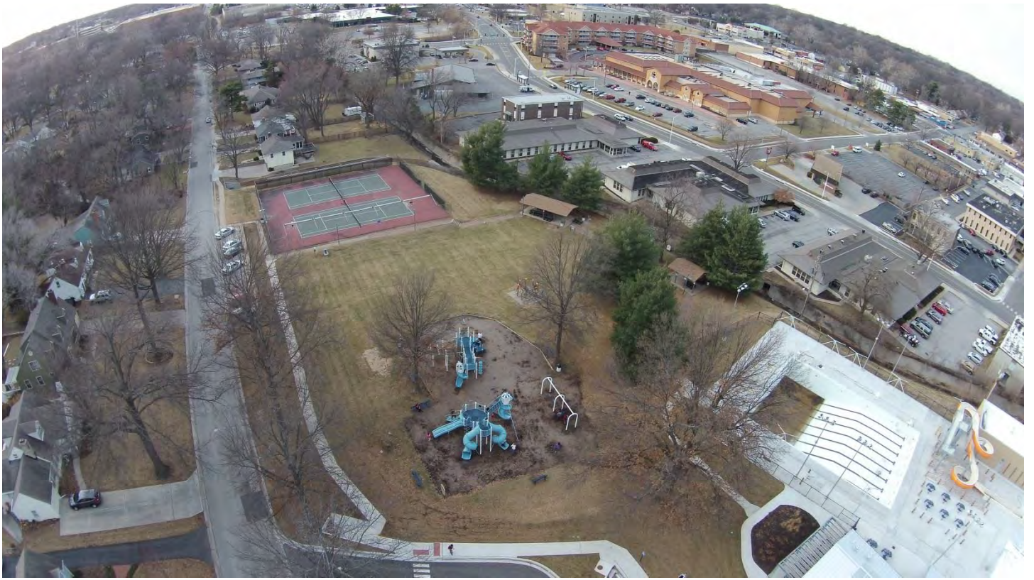
Image 5: Aerial site photo providing a perspective of Andersen Park amenities.
