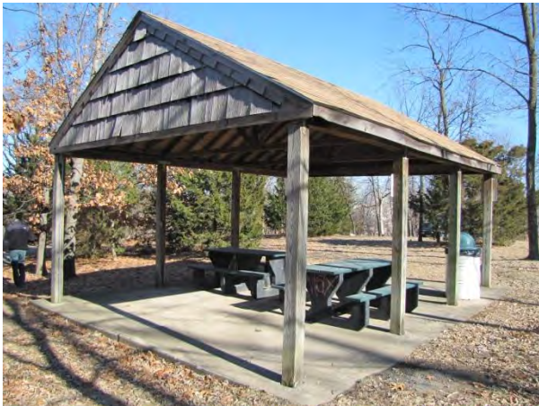
Image 1: The existing park shelter provides locations for small group gatherings.
