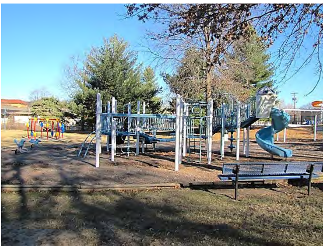
Image 3: Existing playgrounds on site are in need of replacement and surfacing to meet ADA accessibility guidelines.
