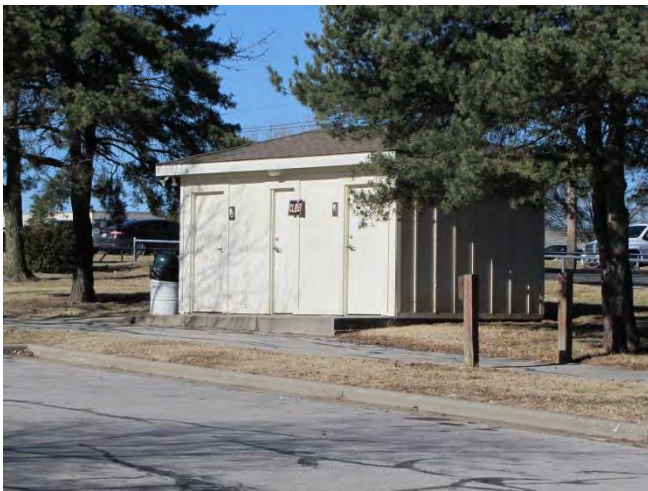
Image 1: Restroom facilities on site support larger gatherings, extended stays, and usage of the park.
