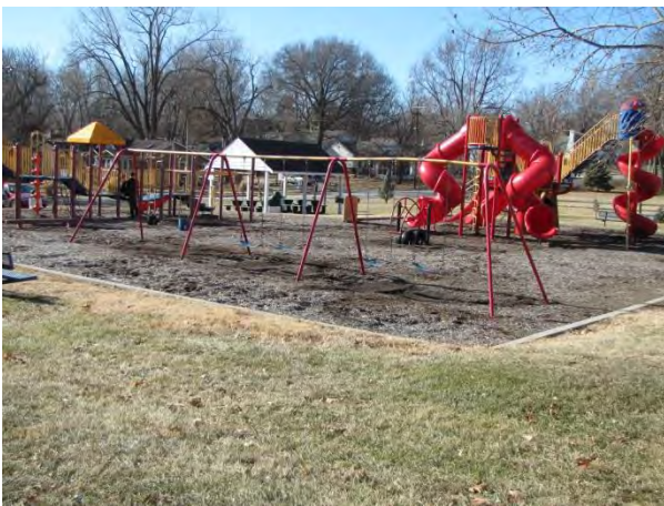
Image 1: Playgrounds and surfacing at Waterworks park are heavily used and need replacement
