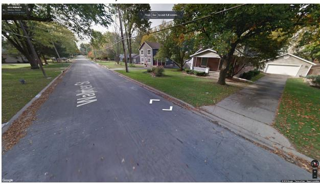
David Schwenk- 5205 Riggs 2017 PCI- 23.9 2008 PCI- 55 Scheduled for Mill & Overlay in 2017. Unsuitable Subgrade.
