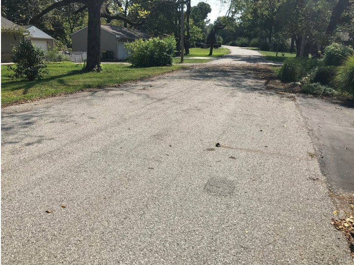
Looking south toward 51st Street
