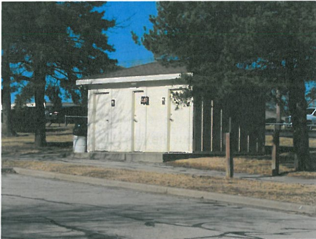
Image 1: Restroom facilities on site support larger gatherings, extended stays, and usage of the park.
