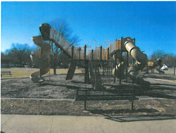
Image 1: Playgrounds and surfacing are in need of replacement to meet current ADA standards.
