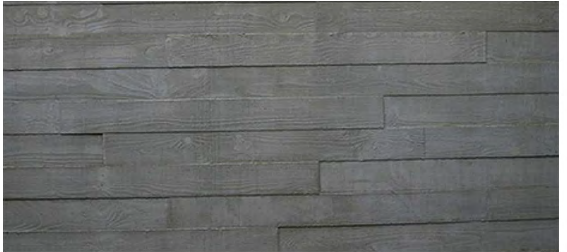
CONCRETE WITH APPLIED COLOR STAIN
