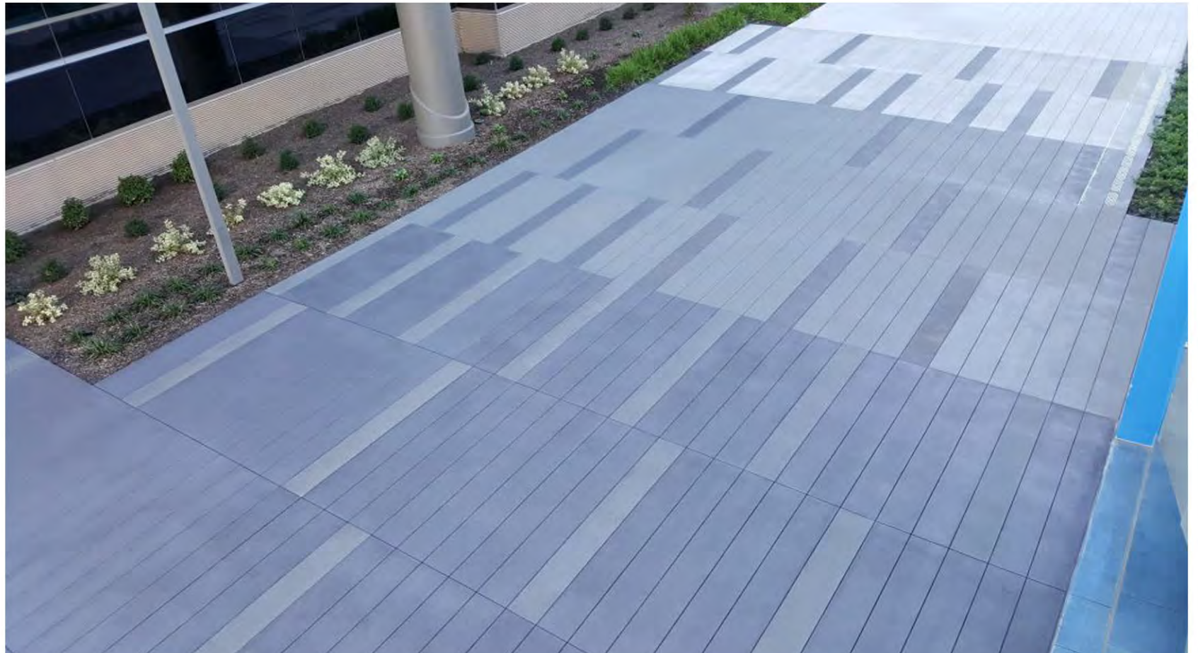
CONCRETE WITH APPLIED COLOR STAIN
