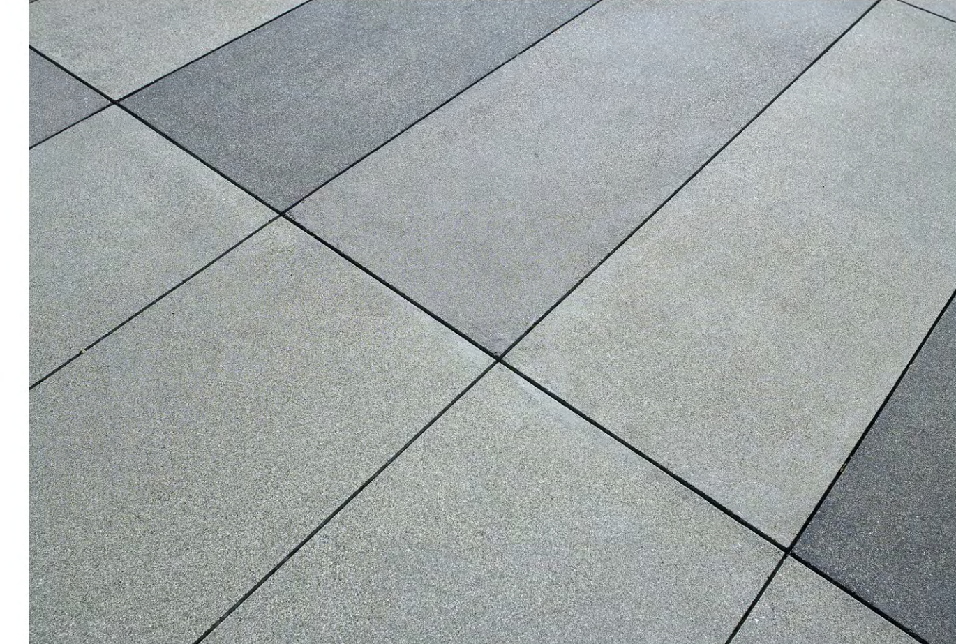
INTEGRAL COLOR CONCRETE - SANDSTONE FINISH
