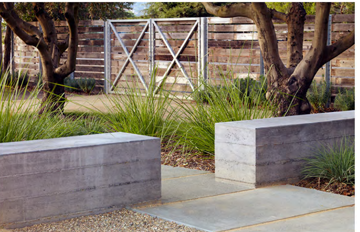
BOARD FORMED CONCRETE WALLS
