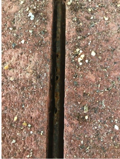
Current concrete joint with metal oxidizing; original concrete joint void former
