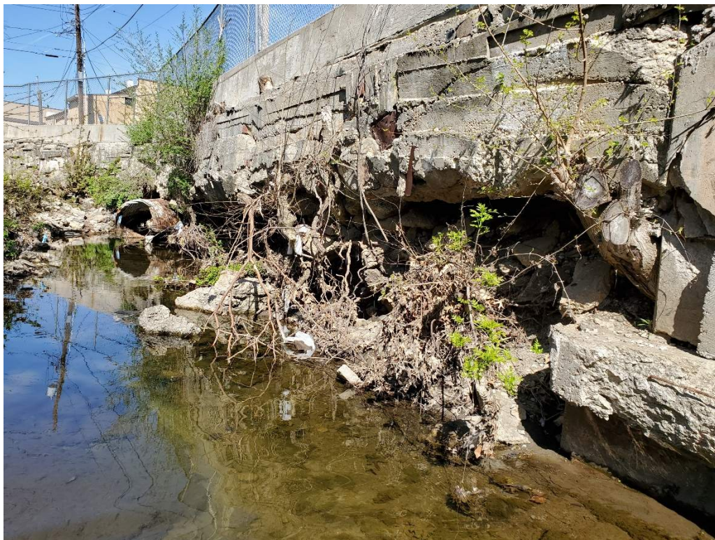
Figure 3: Looking west at prior channel lining/retaining wall and upstream of creek.
