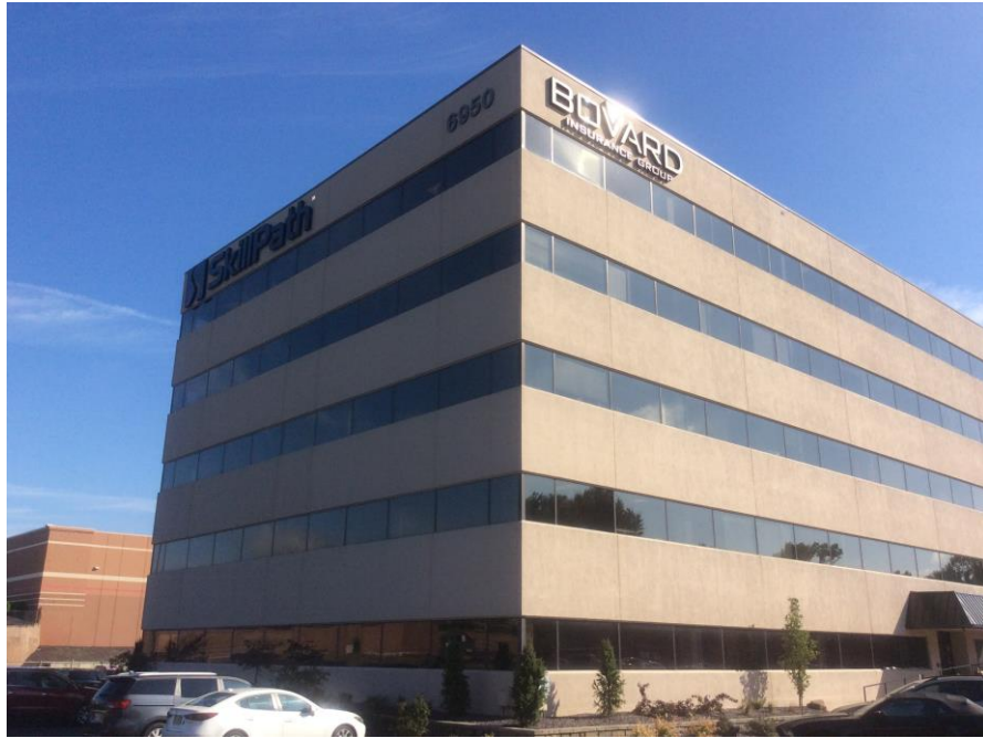
West Side and South Side of Building B - 6950 Squibb Road
