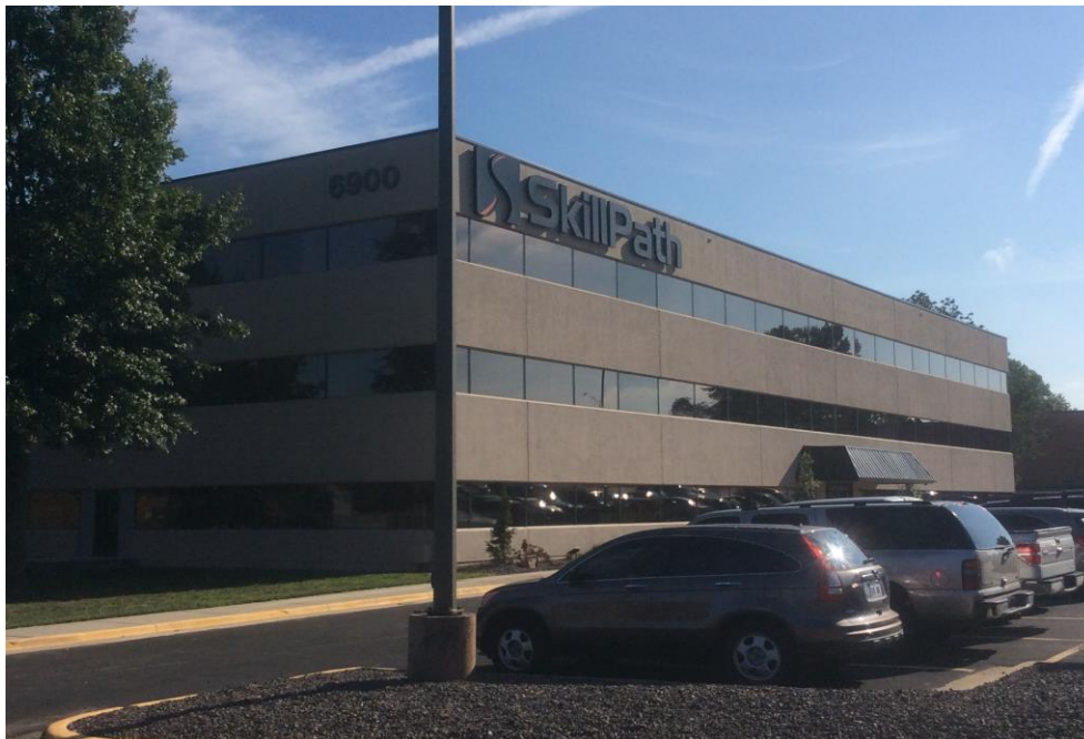
West Side and South Side of Building A - 6900 Squibb Road
