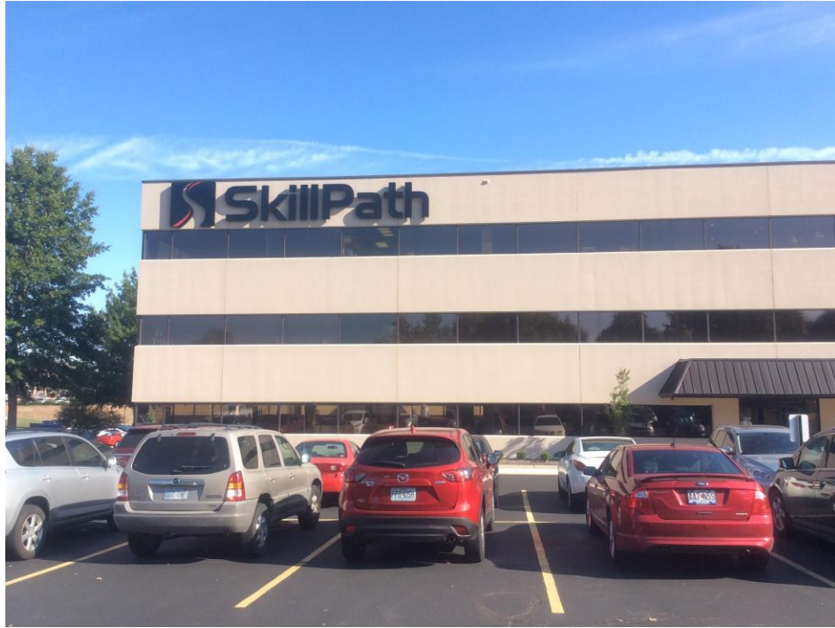
South Side of Building A - 6900 Squibb Road
