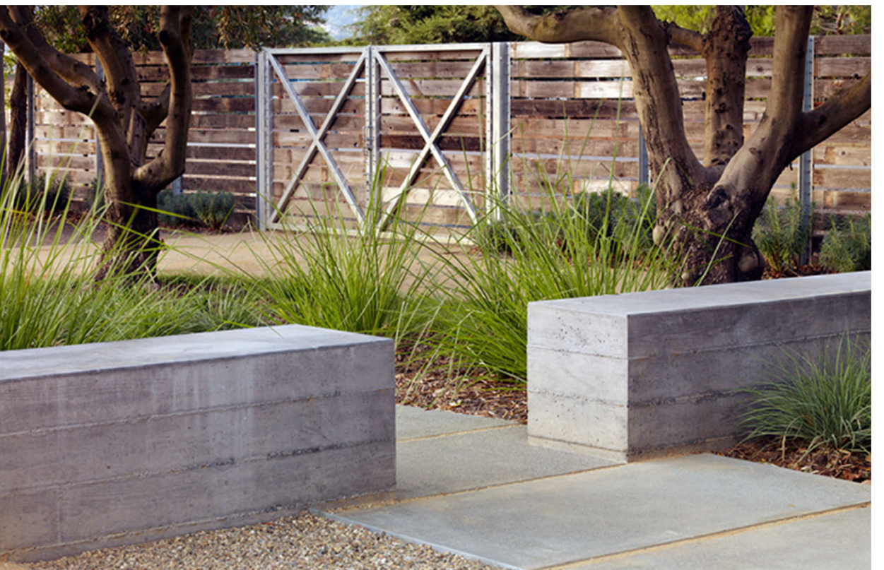
BOARD FORMED CONCRETE WALLS
