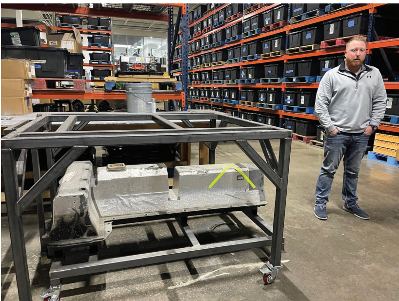
Figure 1. Hybrid battery in outer casing; warehouse shelving with battery components in background.
