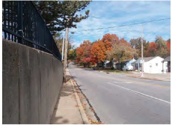
ISSUE: Sidewalk Width and Setbacks on Lamar north of Johnson Drive. Inadequate sidewalk width, back of curb location, horizontal slopes, a vertical wall, and encroaching pole make this sidewalk inaccessible to many users.
