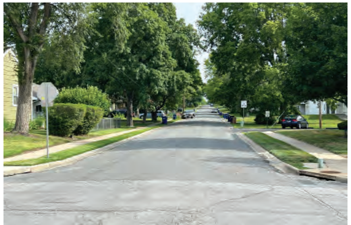
Woodson Road. Good north-south continuity and access to destinations make this a good candidate for adaptation as a bike route.
