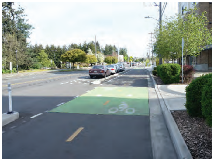
Cycle track. This facility is protected by a raised curb and parallel parking.
