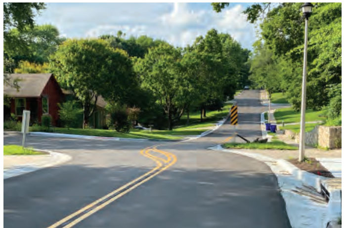
Chicanes or street realignment at specific locations. Goodman Street in Merriam, KS)
