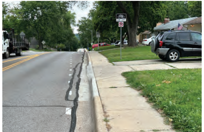
Lamar Avenue Bike Lane. Bike lane is discontinuous at signalized intersections to make space for a left turn lane. Relatively narrow, back of curb sidewalk is typical along this major north-south corridor.
