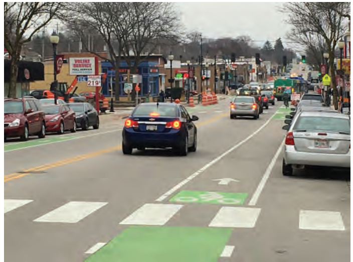
Enhanced Bike Lane. Green paint at the beginning of blocks and at conflict points increase the visibility of the bike lane to both motorists and bike lane users.
