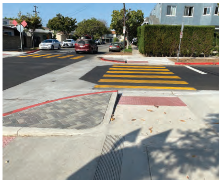
High visibility crosswalk. Crossing installation in Culver City, CA. Wide continental crosswalk striping and directional ramps make this design very comfortable for pedestrians.
