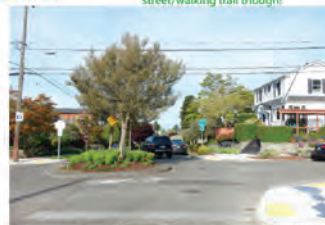
Local street signed as a "neighborhood greenway" with circle to slow traffic Low chance but could do narrowing at entry, intersections to slow traffic
