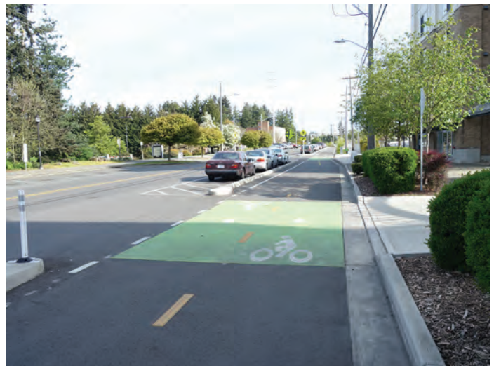
Cycle track. This facility is protected by a raised curb and parallel parking.
