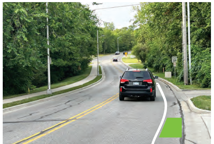
Shared Use Directional Sidepath. In this setting on Foxridge Drive, the existing sidewalk permits northbound only bicycles as well as pedestrians, with an on-street bike lane in the opposing direction.
