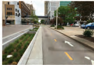
Two-way protected bike lane with a curbed barrier
