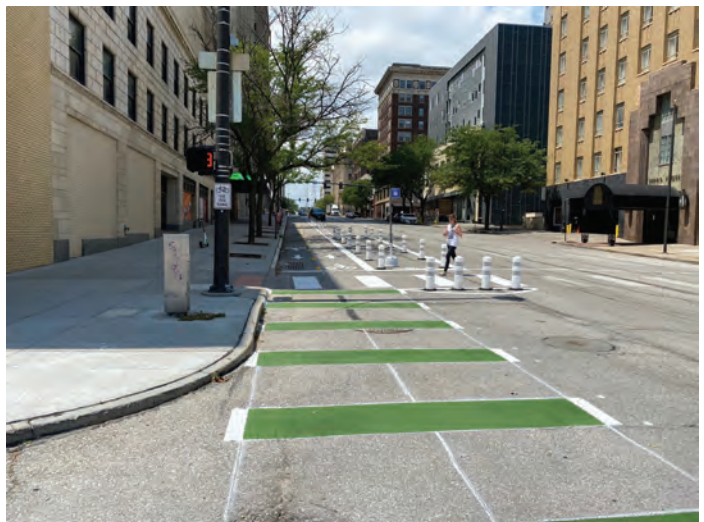
Cycle track. This installation is designed as a pilot project using flexible delineators. Note the "continental style" crossing markings in green..
