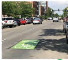
Shared lane marking (sharrow) 6
