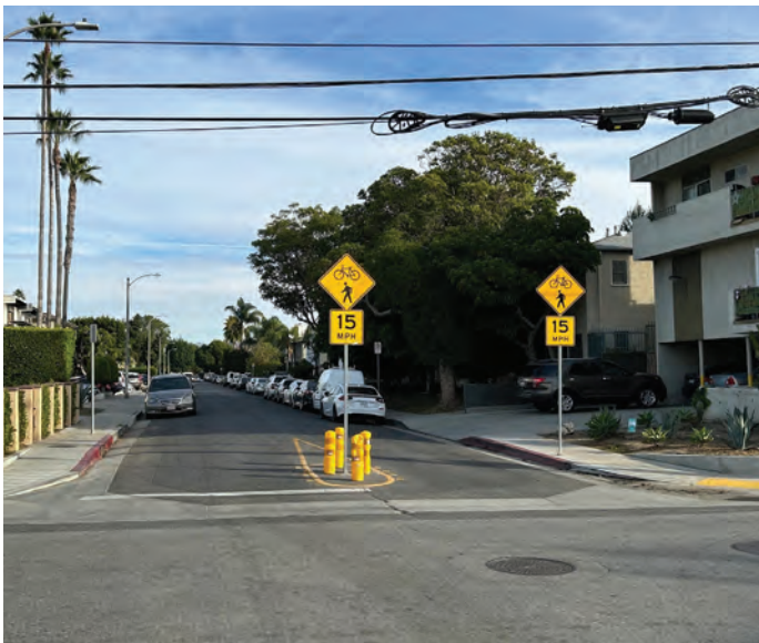
Painted entry median with delineators and signage. This highly cost effective design is in common use in Los Angeles.
