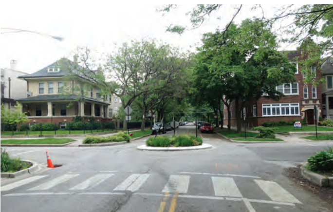
Mini-roundabout. Example from Ravenswood neighborhood in Chicago.
