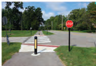
Sidepath with grass separation from roadway and clear driveway and street crossing definition
