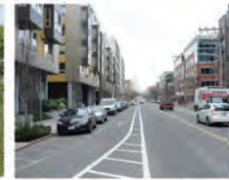
Bike lane with cross-hatched buffer adjacent to travel lane 8
