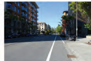
Conventional bike lane adjacent to travel lane Have this - paint alone doesn't work here 1
