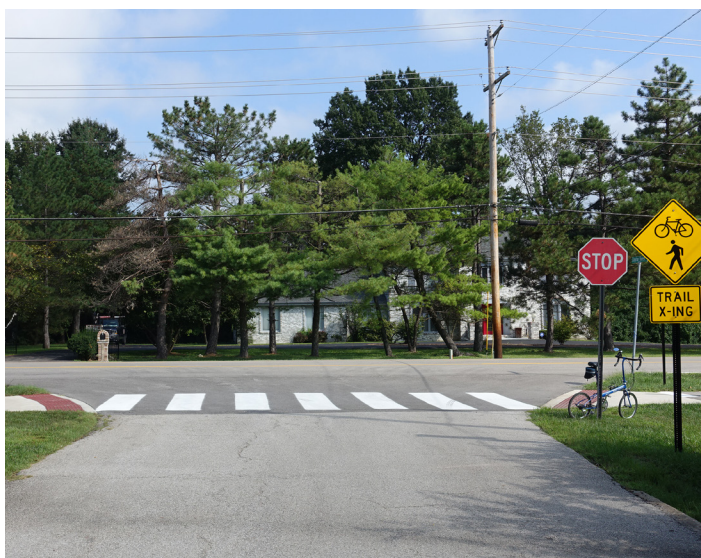
High visibility crosswalk and trail advisory sign, Clayton Road, Saint Louis County, MO
