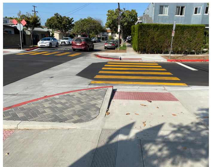
High visibility crosswalk. Crossing installation in Culver City, CA. Wide continental crosswalk striping and directional ramps make this design very comfortable for pedestrians.
