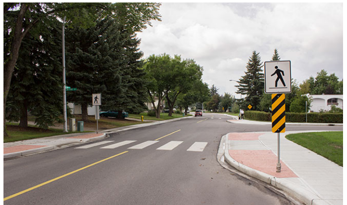
Neckdown. Curb extensions that narrow a street at intersections can moderate traffic speed and reduce pedestrian crossing distance. (Strathcona County, CA photo)
