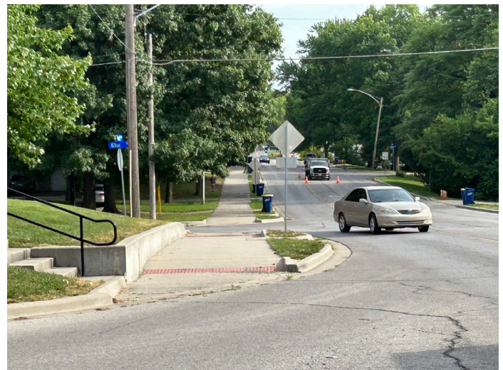
Shared Use Sidepath. Nall Avenue path accommodates travel in both directions. Warning signs for motorists and high visibility crosswalks at street crossings will add to the safety of these facilities
