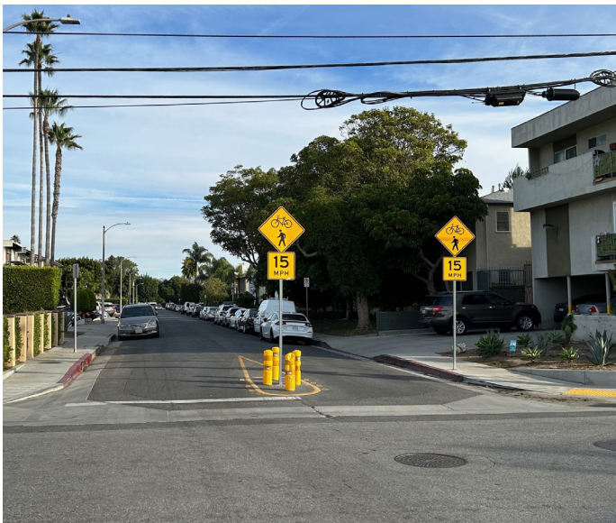
Painted entry median with delineators and signage. This highly cost effective design is in common use in Los Angeles.
