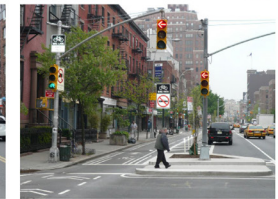
› Parking protected bike lane with raised curb at corners to define parking lane and provide pedestrian protection (one-way) 5 Could work in "front" of diagonal parking along Johnson Drive
